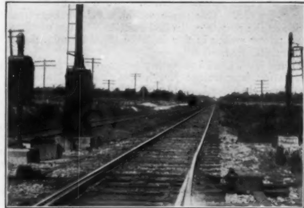
A Remote Control Switch
